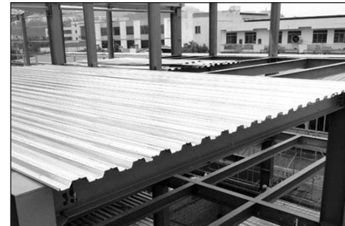
Steel deck and metal roofing
